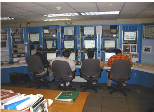
Figure 1: Equipment racks and cramped workspace for operators and support staff.
