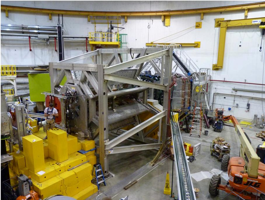
Figure 3.4: Picture of the  $Q_{\text{weak}}$  experiment during the installation. The target is on the left, followed by two lead collimators, one on each side of the man in the photo. A third collimator sits right in front of the large frame in the center of the photo is the QTor magnetic with its eight coils. After QTor on the right three of the eight quartz main detector bars are visible.
