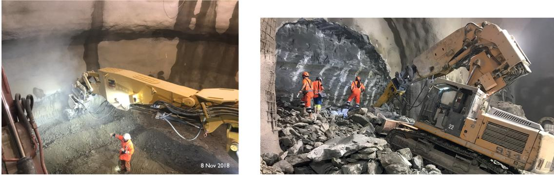
**Figure 8.51:** Left: Roadheader being used for shaft excavation at HL-LHC Point 1. Right: Rockbreaker used for new service tunnels excavation at HL-LHC Point 5 (Credit: Z. Arenas).
