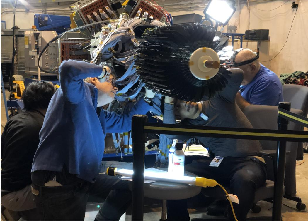
FIG. 68: Cabling work while installing the RTPC in the CVT cart.
